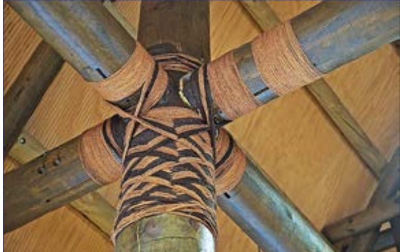
Lalava, the craft of binding buildings with sennit rope made from coconut fibre. These bindings in the Fale Pasifika at the University of Auckland were woven by Sopolomelama Filipe Tohi, a Tufunga Lalava (master craftsman).
