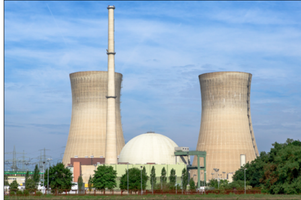
The Grafenrheinfeld nuclear reactor, in the spherical building, with its distinctive cooling towers, Germany, 2013. By Avda, CC BY-SA 3.0.
